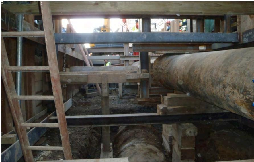
Figure 1 Some utility mains exposed beneath street level
